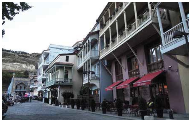
Rebuilt houses in Abano Street, next to the famous sulfur baths in the Old Town.
