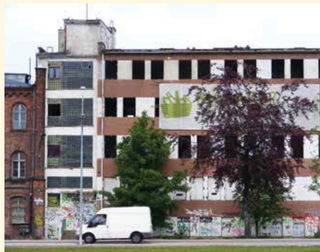
Former Telephone Exchange building (175A) in 2016, Gdańsk Shipyard.
