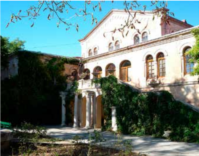
The museum building in the Chersonese, in 2010. In 2013 the Tauric Chersonese National Museum Preserve was UNESCO-listed.
