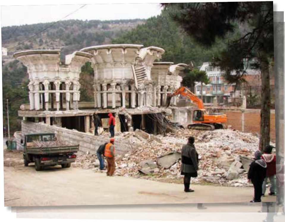
The Palace of Poetry is demolished.
