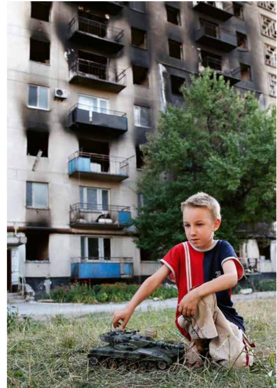
Burned residential apartment building in Luhansk, July 28, 2014.
