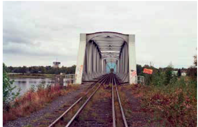
Haparanda–Tornio double gauge rail across the Torne River, looking towards Sweden from Finland.
