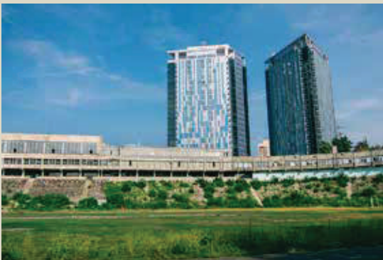
The Burevisnyk Sports Complex was badly damaged during the major offensive by Russian troops. A heavy air raid on March 5, 2022 caused the roof to collapse. It is Valerij S's favorite place.
