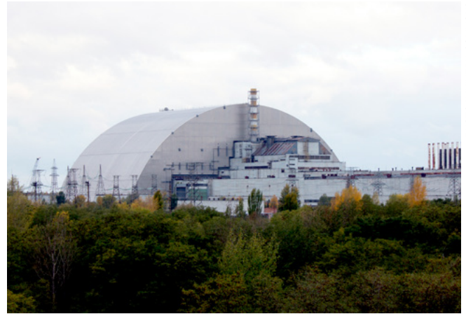
The New Safe Confinement in final position over reactor 4 at the Chernobyl Nuclear Power Plant, 2017.
