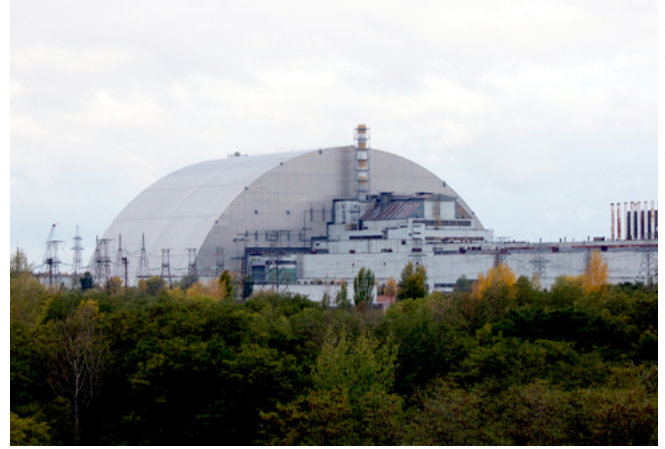
The New Safe Confinement in final position over reactor 4 at the Chernobyl Nuclear Power Plant, 2017.
