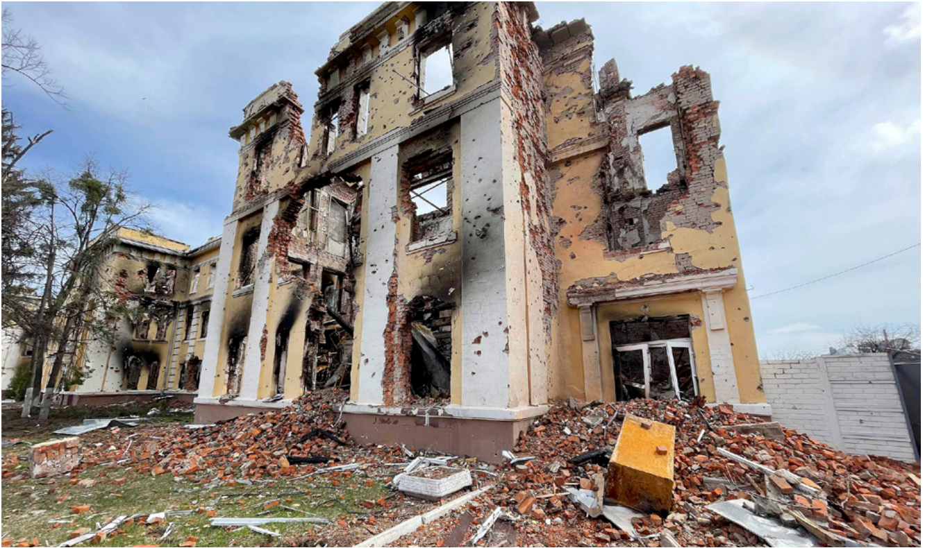
The aftermath of a Russian bombing of a school in Kharkiv, Ukraine in February 2022. An estimated 1 700 schools have been damaged or destroyed in Ukraine since the war started, leaving one in every third child unable to attend school at a full time basis. PHOTO: AMNESTY INTERNATIONAL
