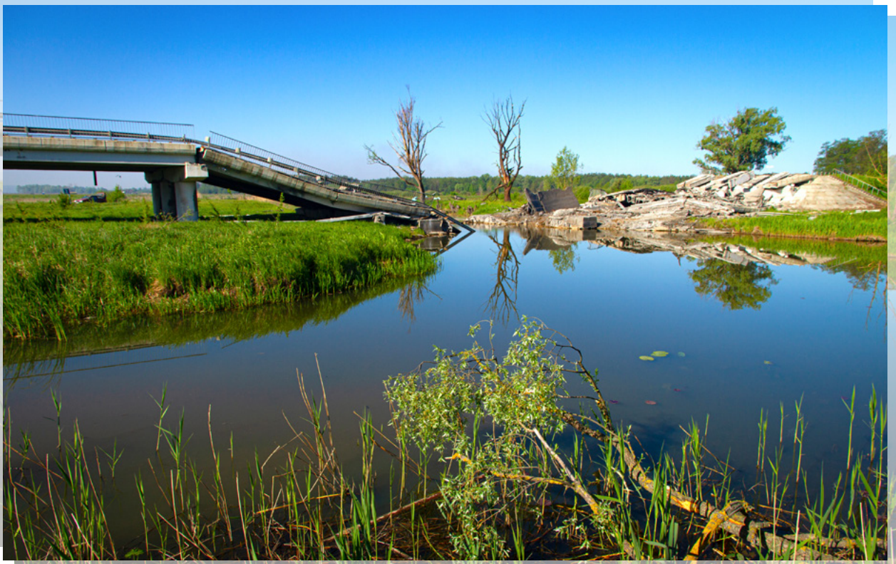
Destroyed bridge on the road to Chernobyl.
